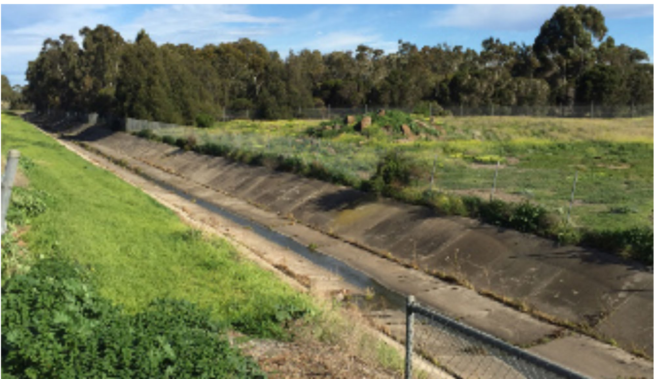
Figure 5 – Upper Stony Creek prior to transformation (source Greenfleet)
